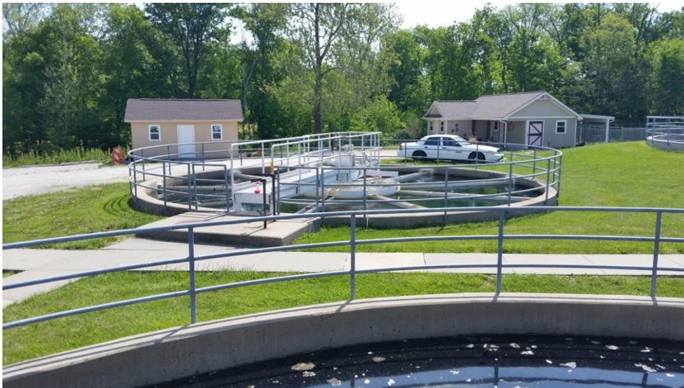
**Figure 4.13 West Basin with a Submerged Collection Pipe**
