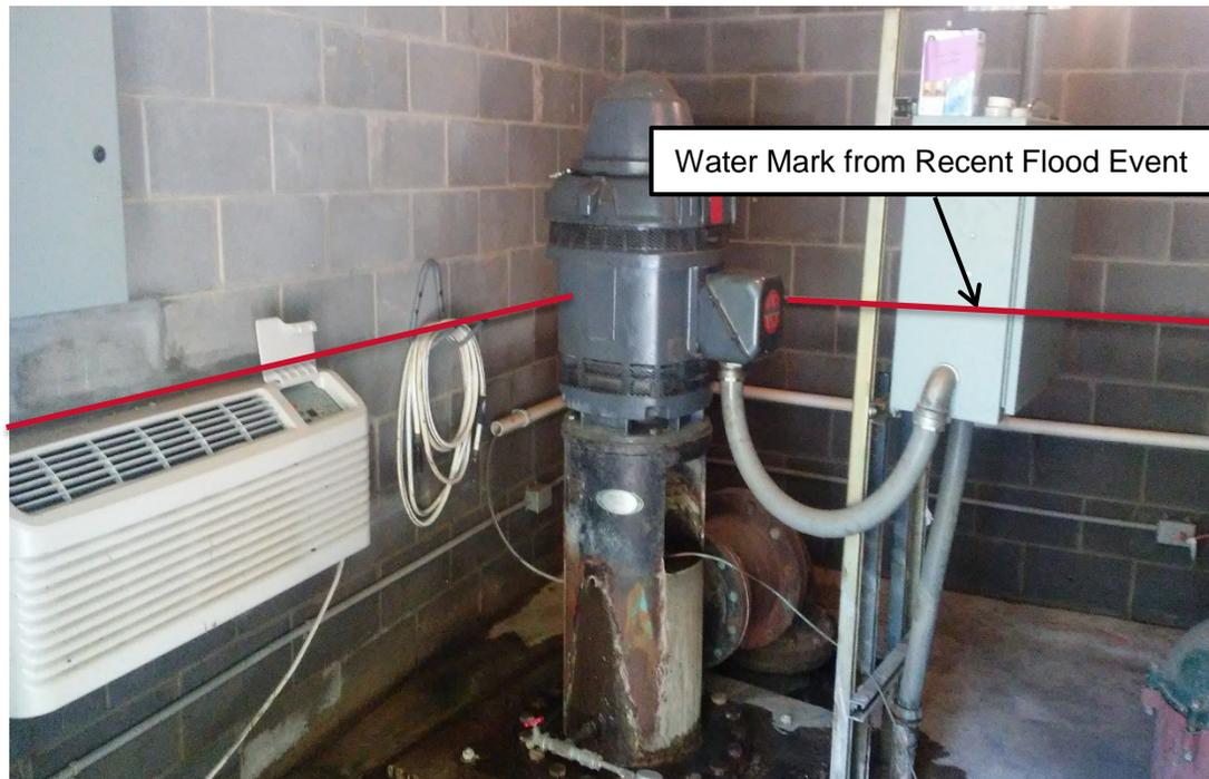
According to City staff, the vertical turbine pump has a maximum available capacity of 1,450 gpm (2.09 MGD) this is the firm and maximum capacity of the pump station. This capacity is 286 gpm less than the WTP current design capacity of 2.5 MGD. Although the pumping capacity is limited, the vertical turbine pump does provide
